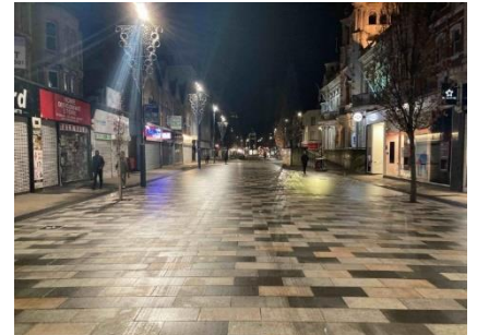
Image 1: New Granite Paving, High Road, Ilford
