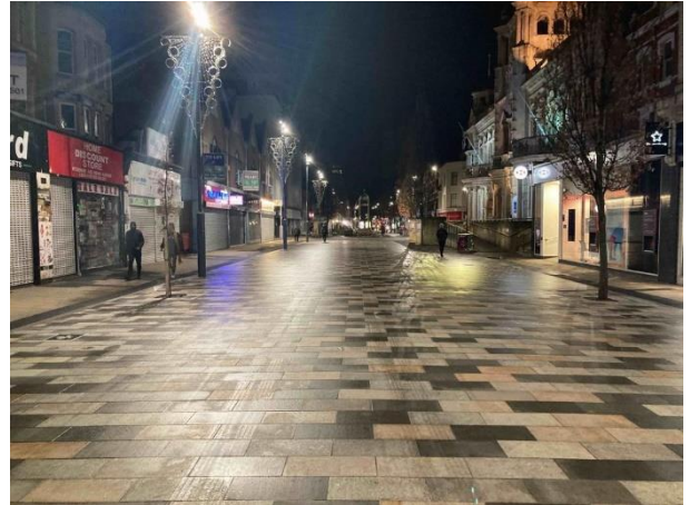
Image 1: New Granite Paving, High Road, Ilford
