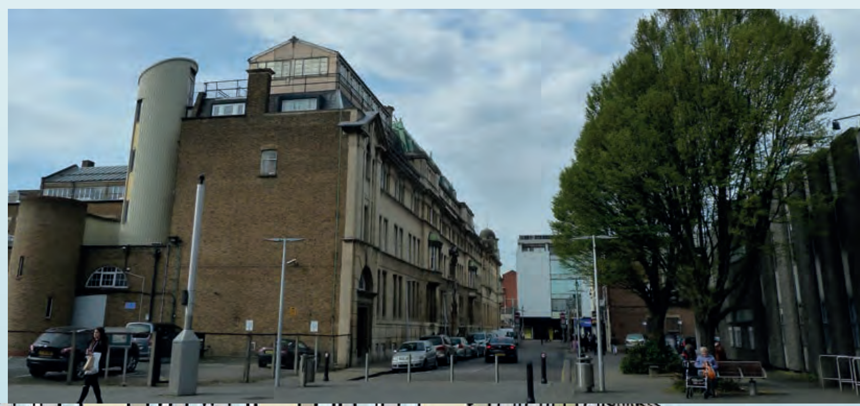
The existing view along Oakfield Road with the council car park to the left and Kenneth More Theatre to the right
